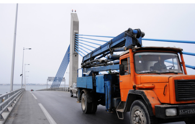
New bridge near Rades industrial zone, Tunisia. © Dana Smillie / World Bank
