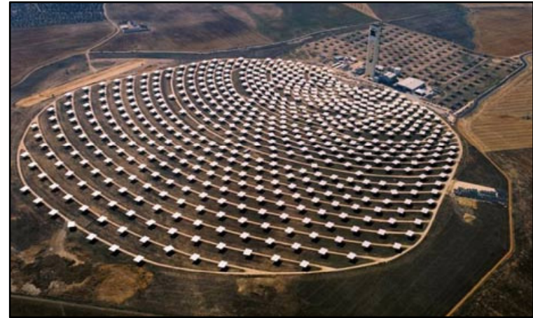
Solar panels in Spain
