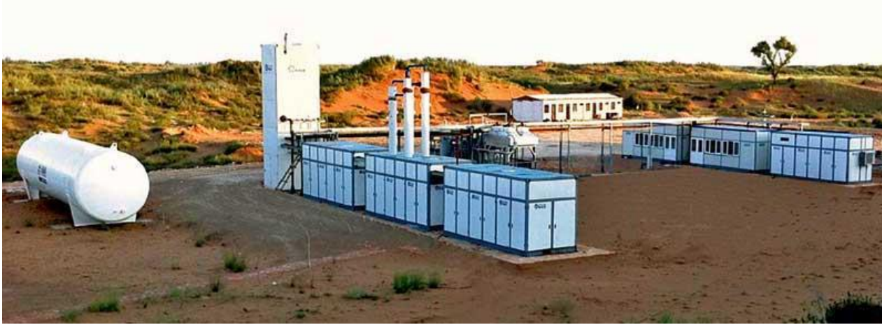
A standard package WSCE MiniLNG-1 at a remote natural gas well site. The capacity is 4,000 US gallons (350,000 ft 3 /d)
